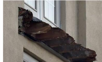
The City, after analyzing that particular failure and the original construction documents and associated structural calculations it was determined that the structural adequacy of the deck as designed and constructed was adequate, yet as shown in the image above there were several detailing issues that led to the structural members decaying and subsequently failing.
